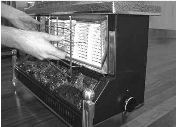
Fig. 2 Remove the Dress Guard.
